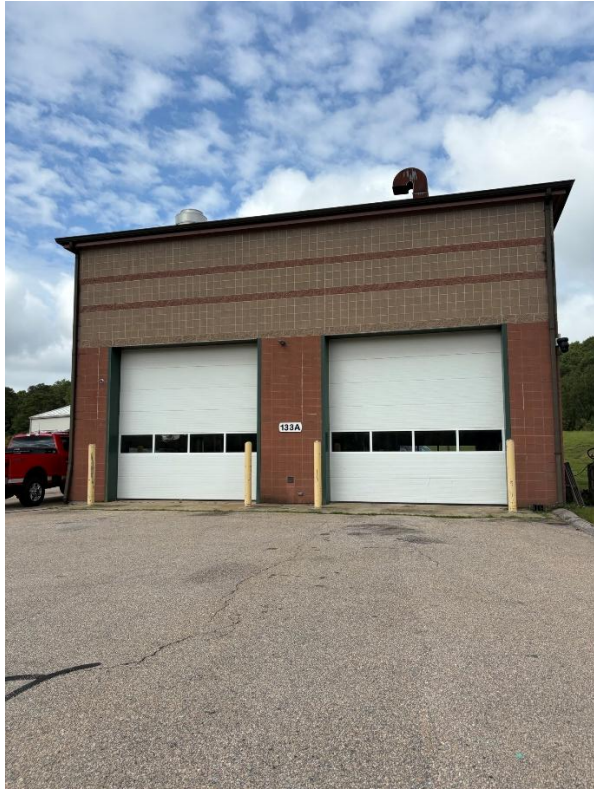
3/4. Mechanic building doors - front
