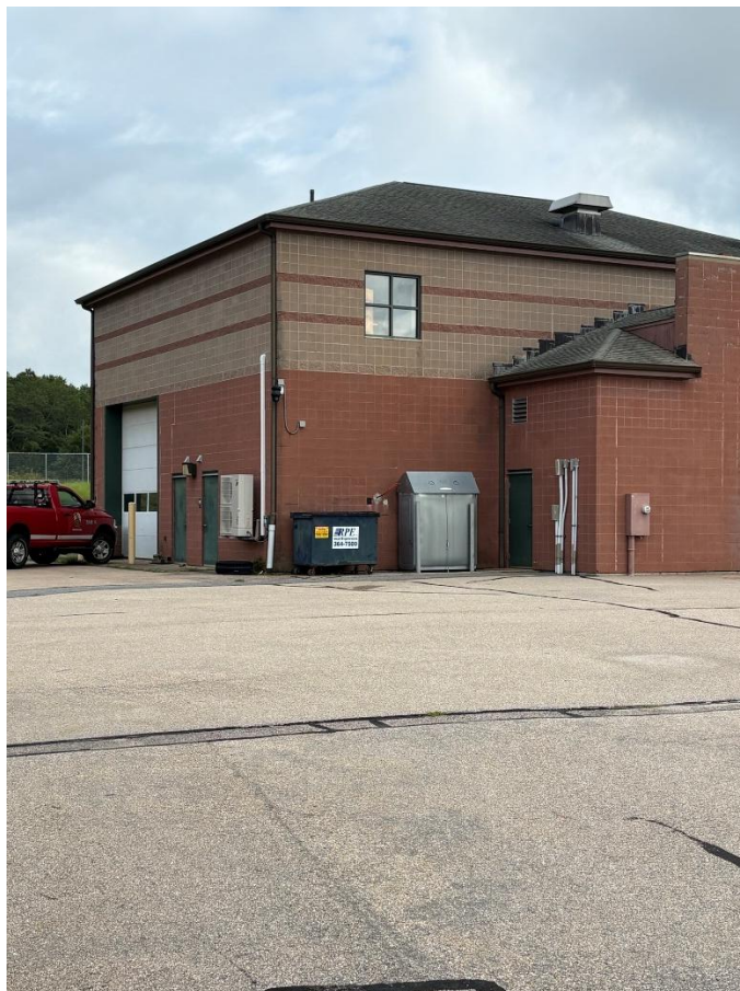
Mechanic building doors - rear
